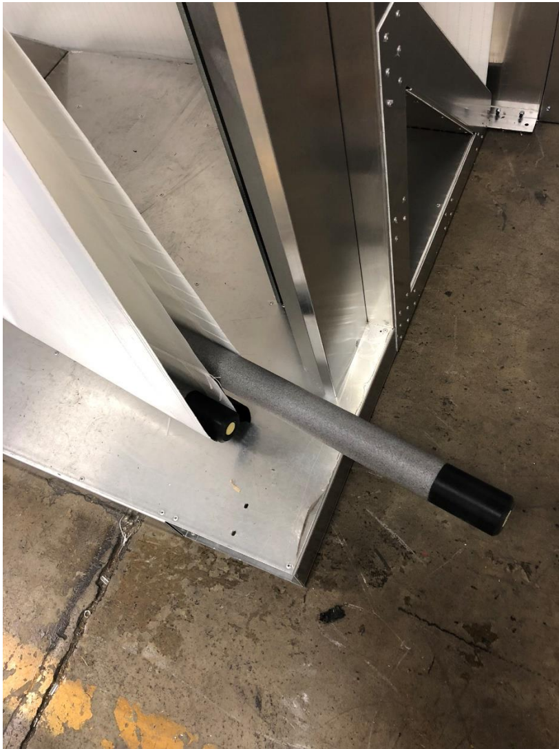
Figure 22: Removal of Tension Pipes
