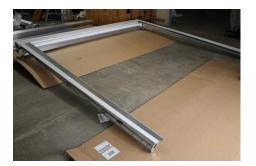
With the door frame lying face down and the tracks aligned with the frame opening, rotate the assembled frame upright by "walking" the legs upright as they are pinned against the cooler wall at the bottom.
