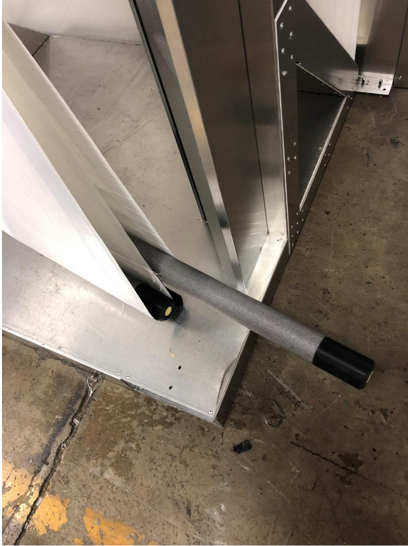
Figure 22: Removal of Tension Pipes
