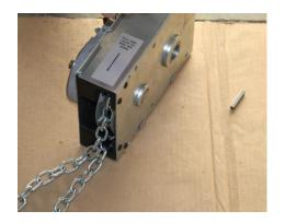
Take the chain hoist up to the shaft protruding from the right side of the door head unit. Rotate the chain so that the keyway in the upper hole matches the keyway position on the shaft. Insert the key from the hardware bag into the keyway of the chain hoist and slide the assembly onto the shaft until it hits the hoist mount on the track.
