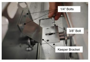
Install the chain keeper approximately 4' off the floor and 6" away from the side of the door track.
