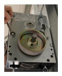
Position the hoist so that the four holes in hoist align with the four holes in the mount and insert the ½"x3" bolts from the door hardware kit in these holes. They must be inserted from the mount side to keep from hitting the cover later. Use the four ½" locknuts to tighten the hoist to the mount.
